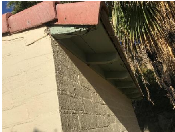
The simple detail of the rafter tails, brick exterior, and terra cotta roof tiles.
