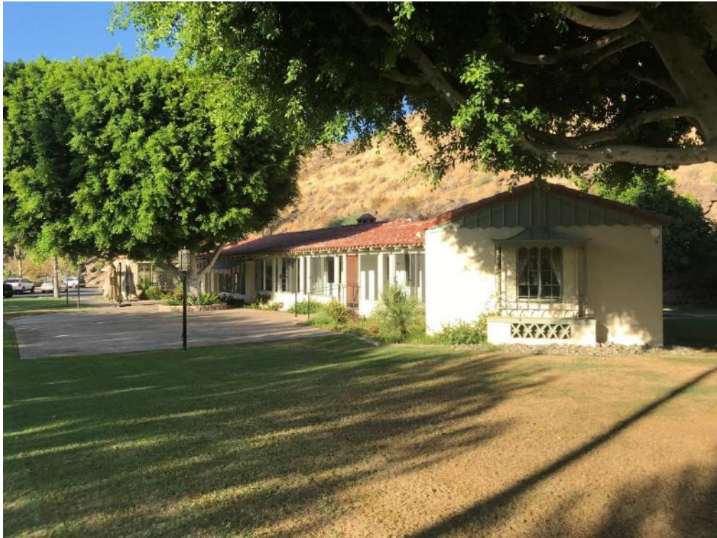
The original bay window and gabled board and batten detailing remain.
